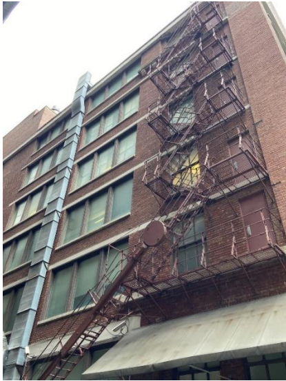
Figure 3: Overall view of the steel fire escape
