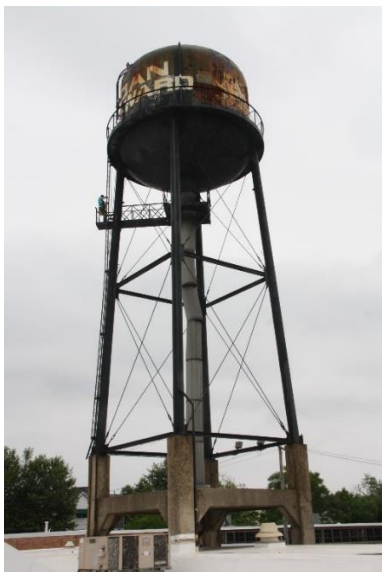
Figure 5: Overall view of the water tower
