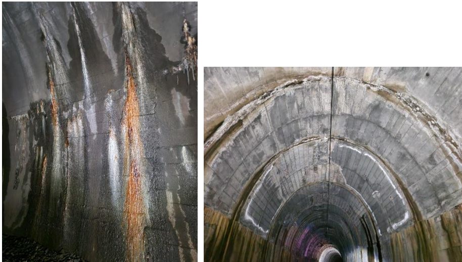
Figure 2: Photographs of the tunnel lining (private archive)
