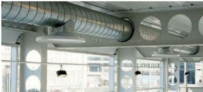
Figure 1: Application example of cellular beams and columns [1]
