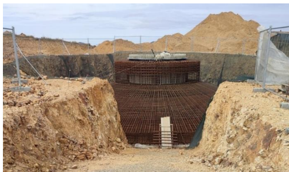
Figure 1: Layout of the reinforcing cage of the wind turbine foundation at the construction site
