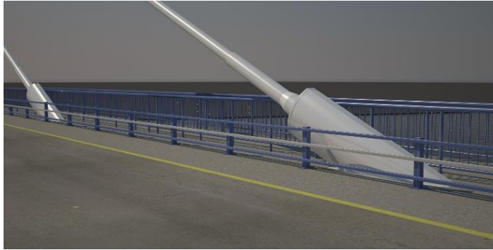
Figure 3: Cable fire encapsulation at deck anchorage
