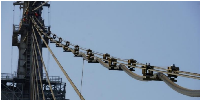
Figure 2: Detensioned cable being lowered on the temporary cables with roller assemblies
