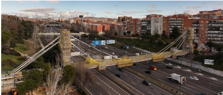
Figure 6: Works being delivered about the main ring road in Madrid
