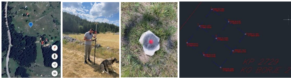
Figure 2: Experimental site and geodetic setup: (a) satellite view of the study location in Vrela, Montenegro; (b) geodetic marking of reference points; (c) marked ground points serving as initial assembly references; and (d) the geometric layout of the steel hall structure with predefined coordinates for columns and beams (source: authors' research)
