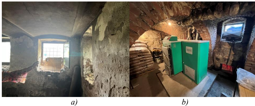
Figure 3: a) low brick vault School buildings in a village Krusevici, and b) pitched-brick vault in a village Mali Crljeni
