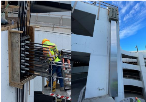
Figure 12: One new anchor block for the vertical external post-tensioning system at the top of the column
