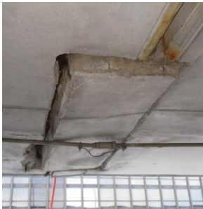
Figure 5: Dropped, rotated, and spalling concrete infill blocks
