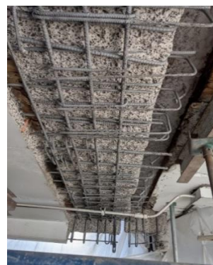
Figure 9: Repair of deterioration of the underside of the ramp slab at the joint between the ramp and the parking deck
