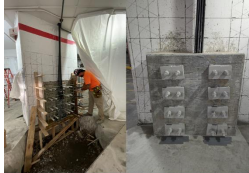
Figure 13: One new anchor block for the vertical external post-tensioning system at the base of the column
