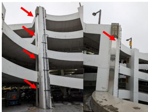
Figure 15: Finished EPT column repair (red arrows) with stainless steel cover protection against UV degradation
