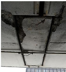
Figure 5: Dropped, rotated, and spalling concrete infill blocks
