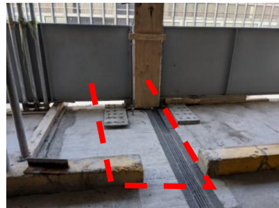
Figure 6: Dropped infill block replaced with monolithic concrete (original position of infill block outlined)
