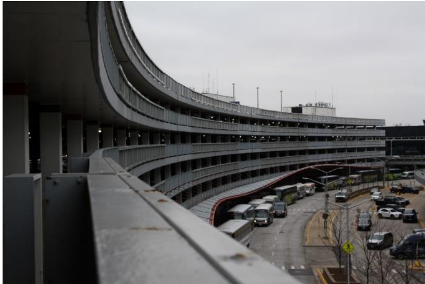
Figure 1: Overall view of the south elevation of the elevated parking structure
