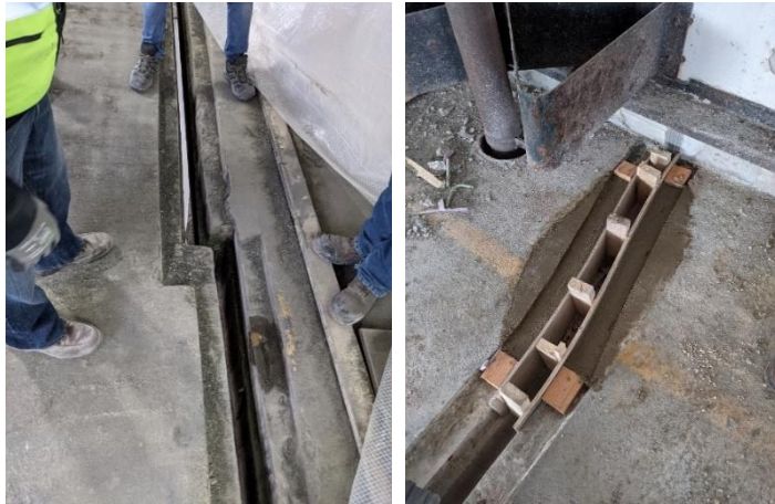
Figure 7: Jog in expansion joint removed to allow for continuous joint seal installation
