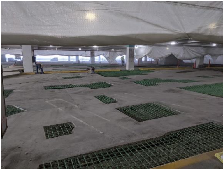
Figure 2: Full depth concrete repair openings in the work enclosure
