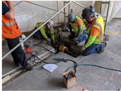
Figure 4: Girder PT restressing
