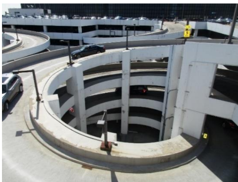
Figure 8: Helical ramp structure
