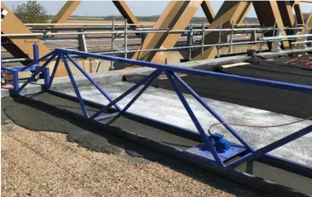
Figure 3: Leveling ruler for overlay INSTALLLEMENT (source Freyssinet)
