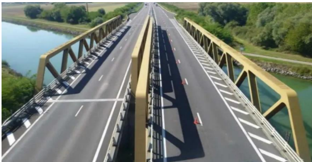
Figure 1: Bridge overview (source Freyssinet)
