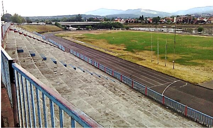
Figure 1: Former appearance of the athletics stadium in Kraljevo
