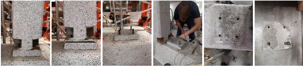
Figure 6: Demounting procedure of the precast column–foundation connection
