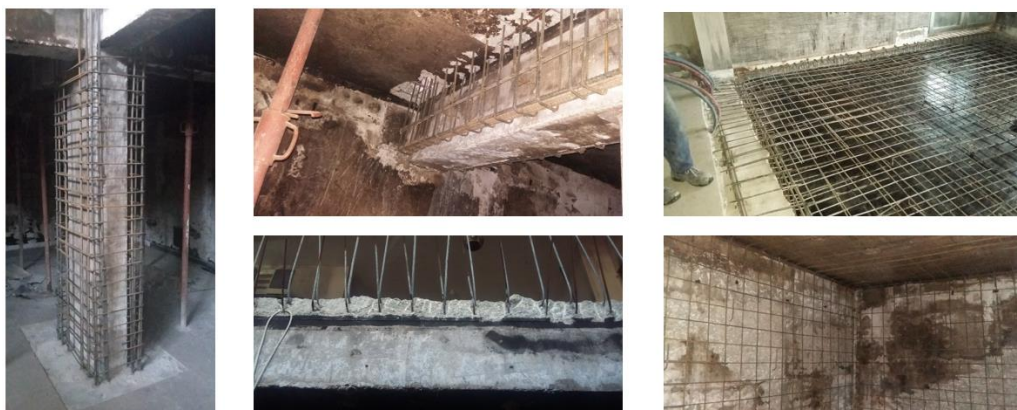
Figure 7: Repair and strengthening of fire damaged RC structural elements
