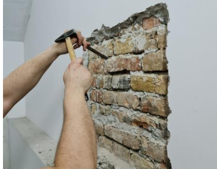
Figure 3: Preparation of the test location
