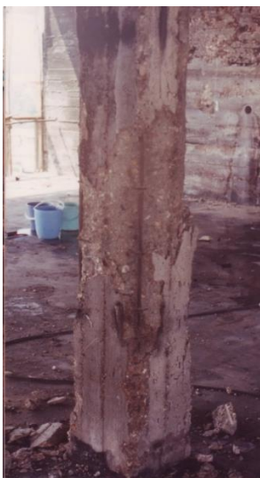
Figure 8: Crack within the concrete of RC columns affected by the fire
