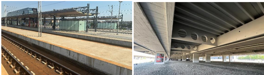
Figure 4: General view of the railway bridge at Novi Beograd, from above and below
