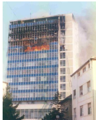
Figure 7: 9th floor affected by the fire
