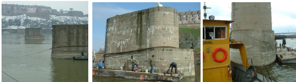
Figure 13: Use of boats and barges to prepare for the inspection of the piers
