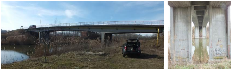
Figure 1: General view of the road bridge over the DTD canal
