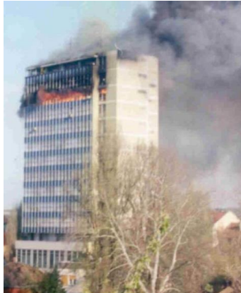
Figure 6: 11th floor affected by the fire
