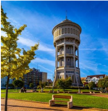
Figure 9: The first water tower built of reinforced concrete in Hungary (1904, Szeged, Hungary)
