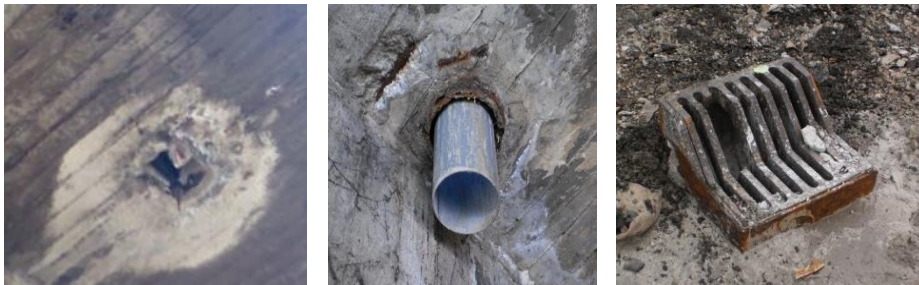
Figure 3: Components of the Gazela Bridge drainage system (drainage openings, outlets, and inlet grates) prior to the 2012 rehabilitation
