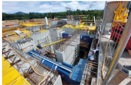
Figure 5: Strengthening and rehabilitation measures applied to the existing reinforced concrete piers, foundations and abutments
