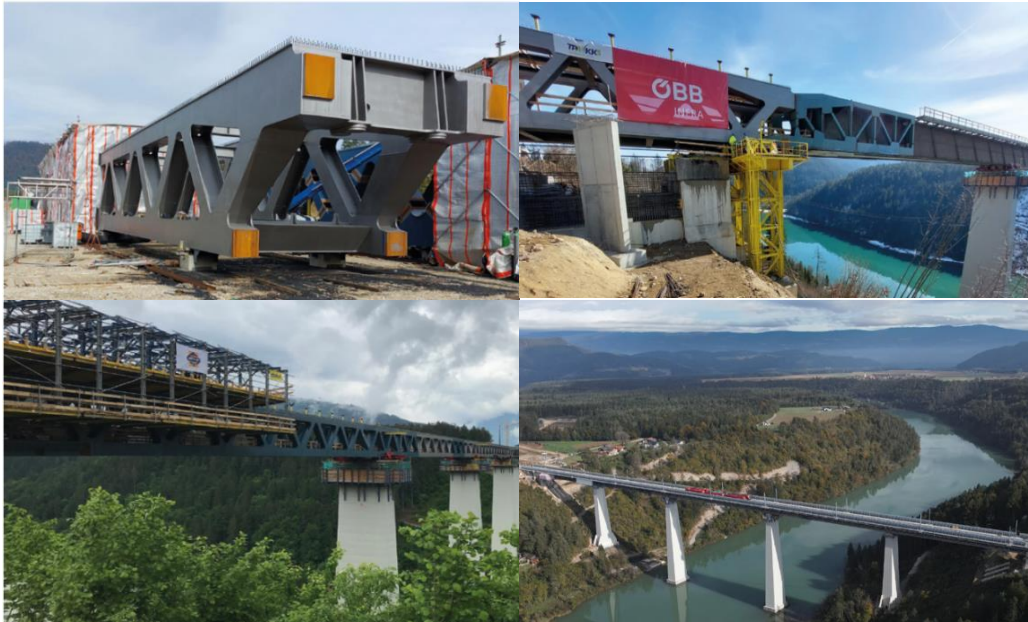
Figure 6: Construction sequence for replacing the Jauntal Railway Bridge by incremental launching and sequential construction of the composite concrete deck slabs on the steel truss system
