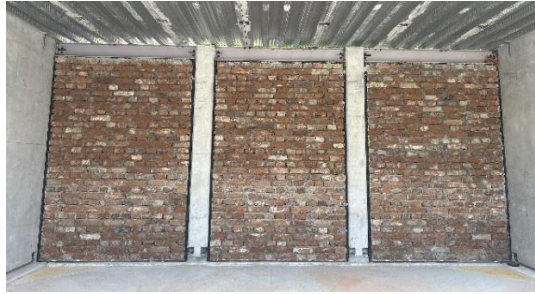
Figure 3: Precast infilled frame in the 3R pilot house
