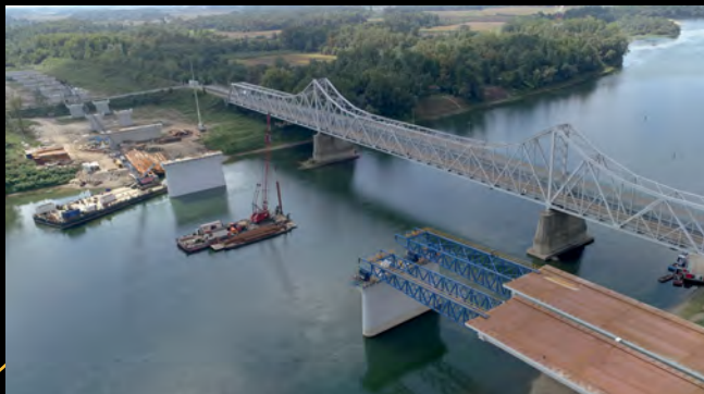
Bridge over Sava River in Sremska Rača
