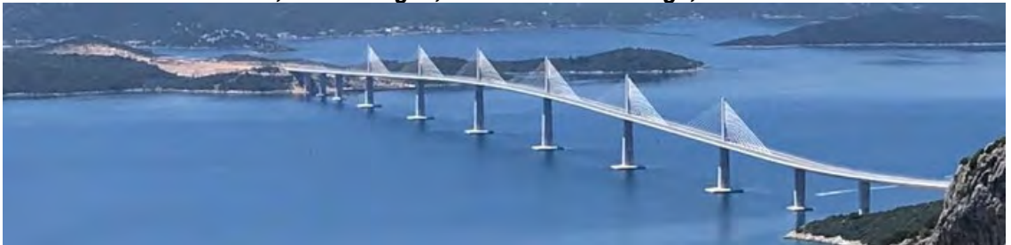
Peljesac bridge with access roads project, L=3940 m, Croatia, with extrados bridge L=2404 m, 6 towers, spans 285 m, piles Lmax=136 m (70% piles are more than 100 m)
