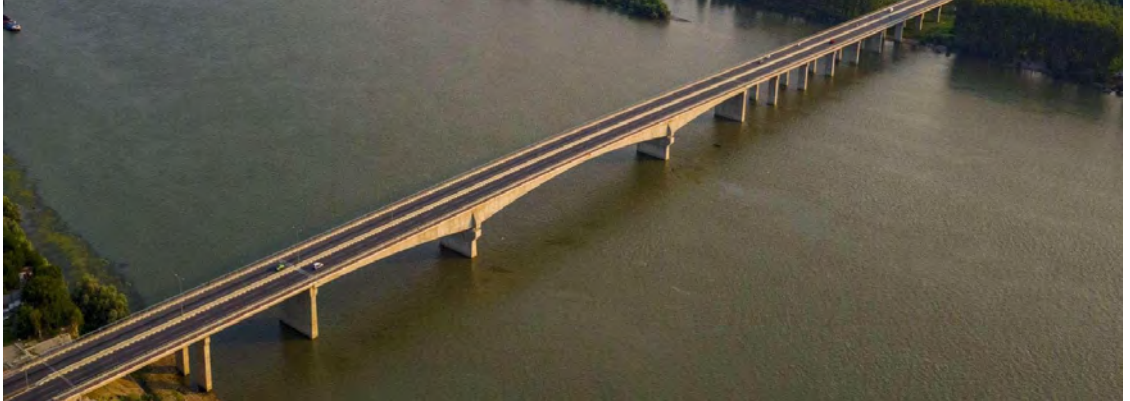
North tangent Belgrade internal ring road, L=22 km, with 1481 m Zemun – Borca, prestressed concrete continuous girder bridge over Danube river
