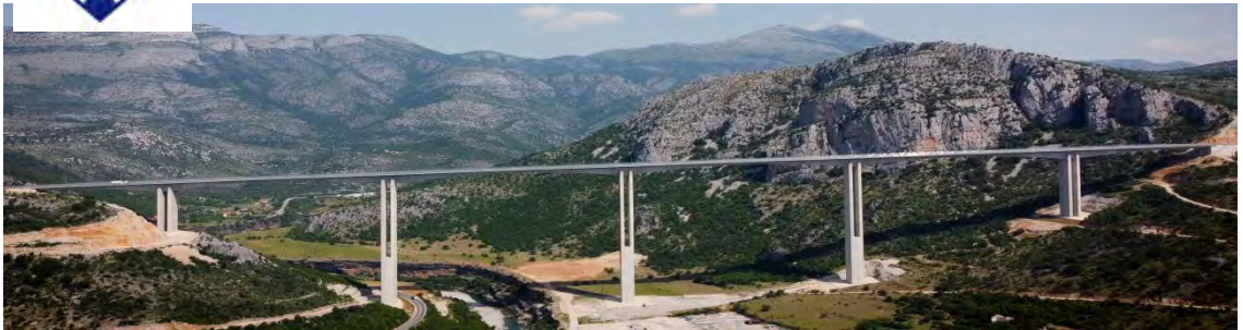
Bar – Boljare highway, section Smokovac – Matesevo L=41 km, Montenegro, 18 km tunnels, 7 km bridges, with Moračica bridge, L=960m
