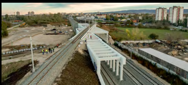
Gallery at km 78+377
