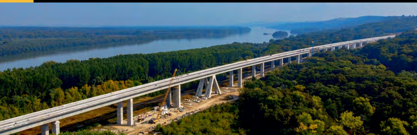
Viaduct Čortanovci at km 59+159,40
